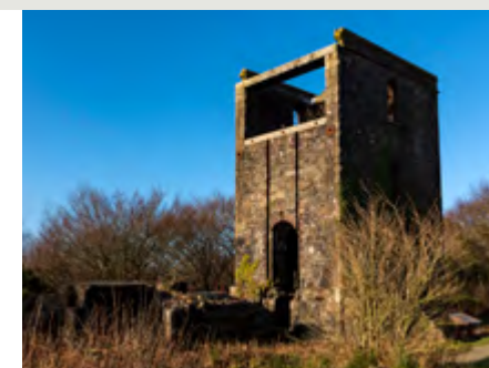
Top Mount Foundry/ Tavistock Iron Works Above Bailey's Shaft engine house, Hingston Down Consols Mine
