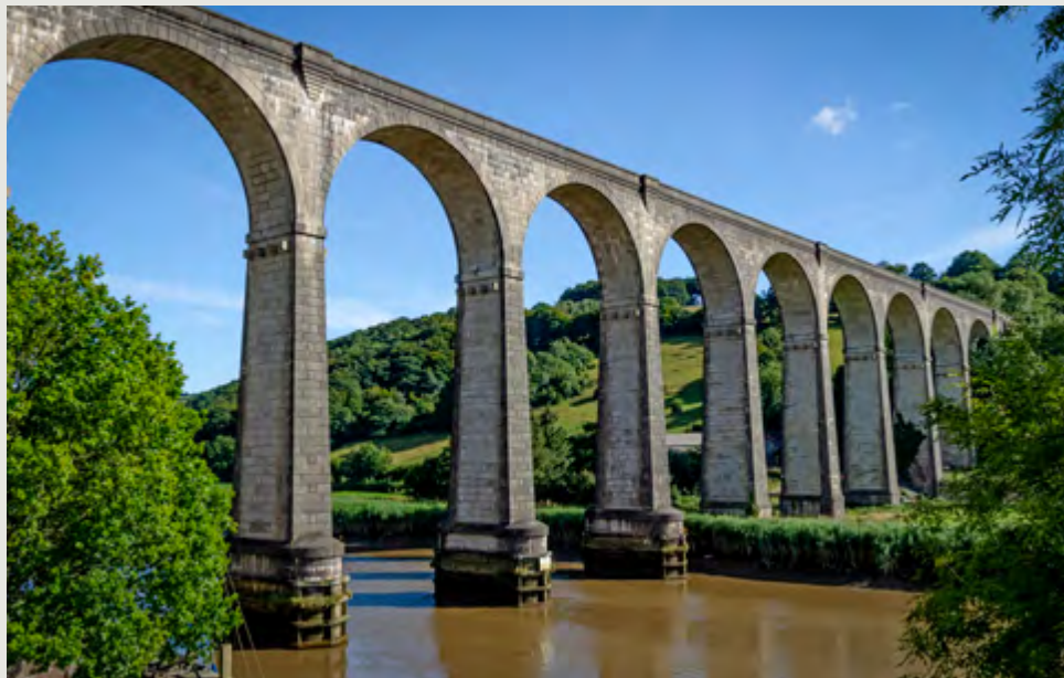
The Calstock Viaduct over the River Tamar
