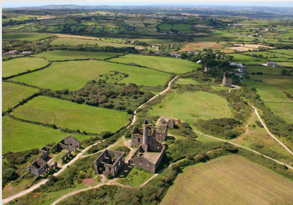
Basset Mines Marriott's Shaft complex on the Great Flat Lode
