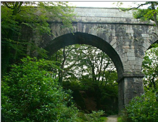
Treffry Viaduct. Photo: Tony Atkin
